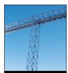
Catwalk Support Towers are custom engineered for height, wind, speed or seismic zone. Freestanding or guyed, with the option to add access bracing, conveyors, spouting and other custom configurations.
