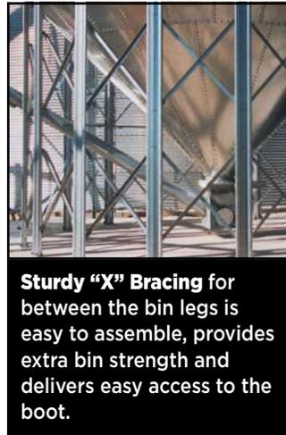
**Sturdy "X" Bracing** for between the bin legs is easy to assemble, provides extra bin strength and delivers easy access to the boot.
