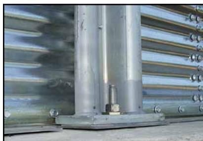
**Anchor Rod/Bolt System** is included on all models. The adhesive or cast-in anchors provided meet new ACI concrete code requirements and help create a strong, weather-tight connection to the foundation, protecting your investment from winds up to 105 mph (169 kph).
