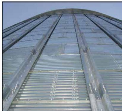
**All-Galvanized Steel** stiffener design carries 100% of the bin's vertical load stresses and leads the industry in strength. Stiffeners are assembled with bolt heads inside bin and flange nuts outside for easier assembly and to minimize interior grain hang up points.
